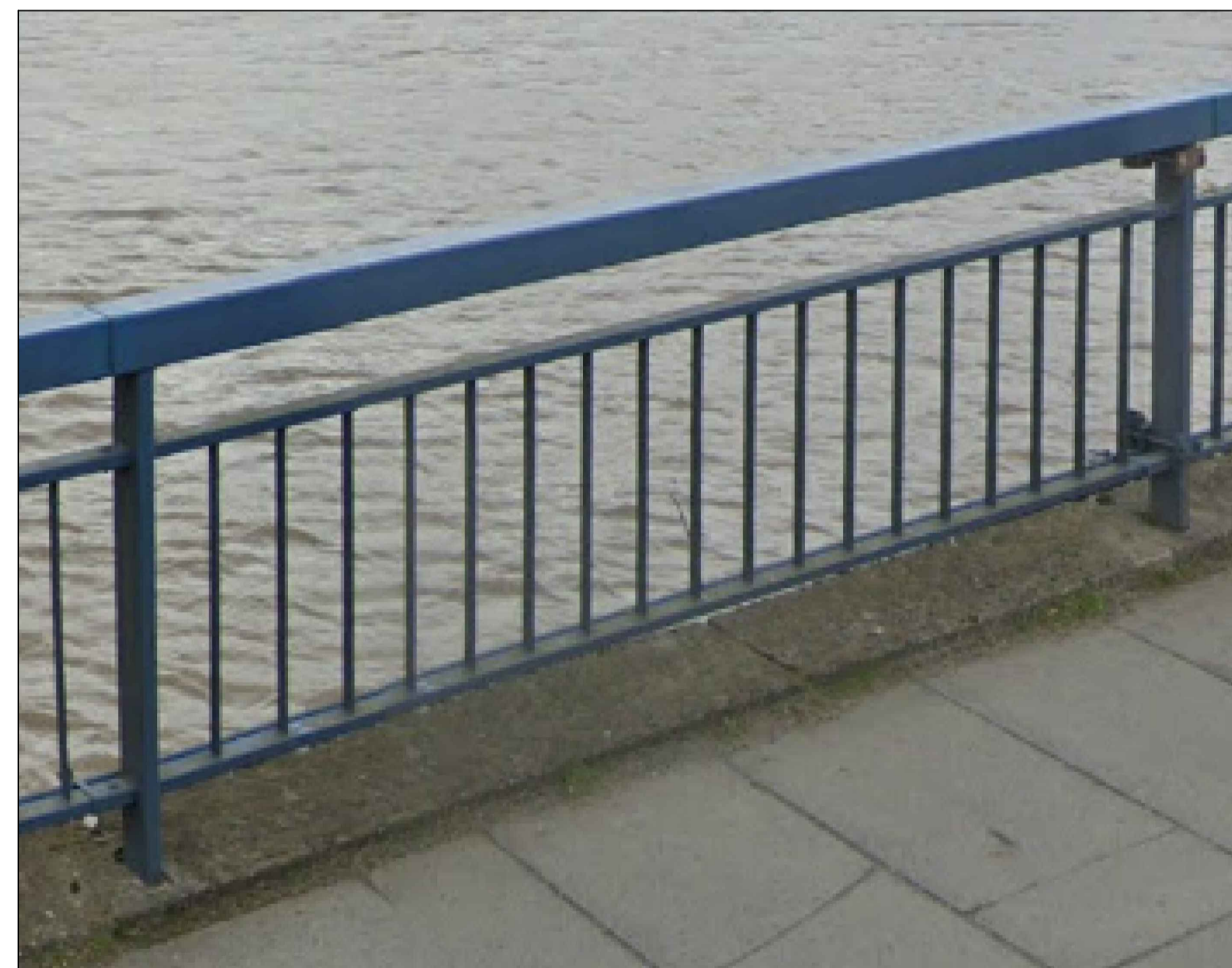
EXISTING PARAPET SAMPLE
