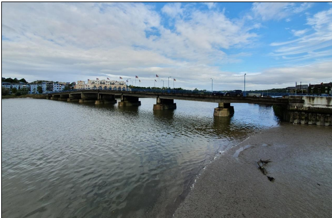
Plate 2-7 Estuary / Tidal River flowing under O'Hanrahan Bridge.
