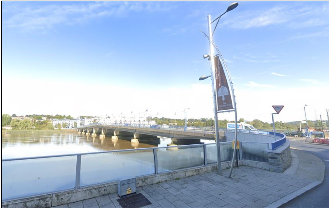
Plate 2-1 New Ross Quay with view to the north. In the foreground are the existing road, footpath and the existing flood defence wall at the south-east corner that is within the proposed development. In background is the O'Hanrahan Bridge. © Google Street View
