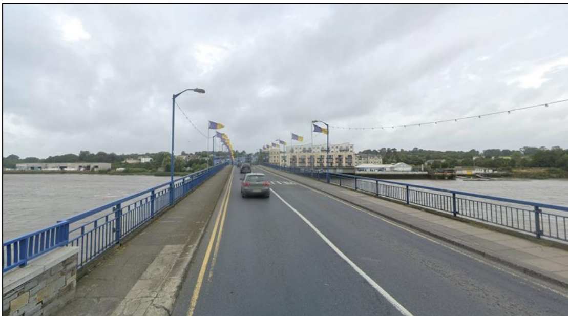
Plate 2-2 O'Hanrahan Bridge with view to the north-west. In the foreground are the existing road of the bridge and the narrow footpaths along the sides that are proposed to be widened as part of the development. The existing parapets are proposed to be replaced. © Google Street View
