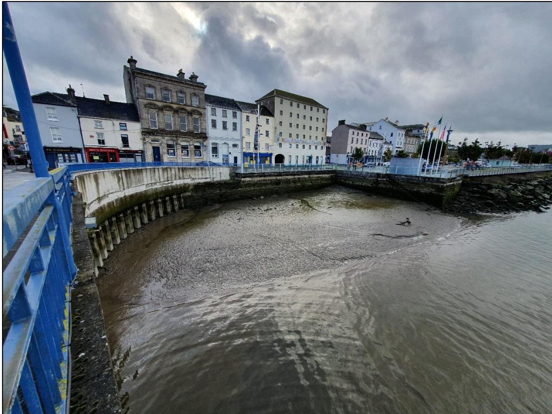
Plate 2-9 Mud Shores, Sea Walls, Piers and Jetties, and Buildings and Artificial Surfaces at the south-eastern corner of O'Hanrahan Bridge.
