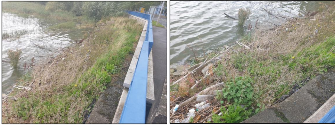
Figure 5: Photos 5 and 6 Shows vegetation on rock protection at O'Hanrahan's Bridge
