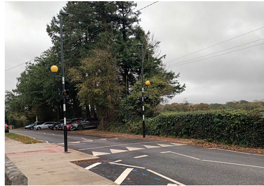
Zebra Crossing - Belisha Beacons with Integrated Street Lighting mounted on top
