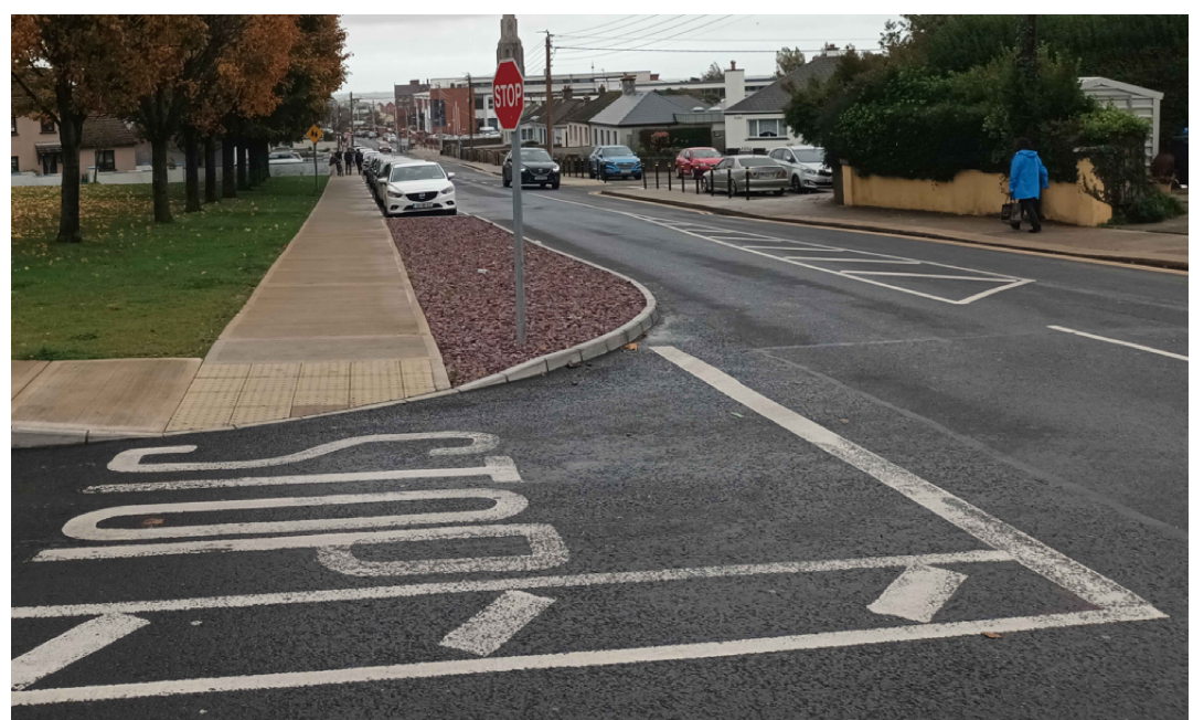
Example of decorative stone use to backfill when reducing corner radii
