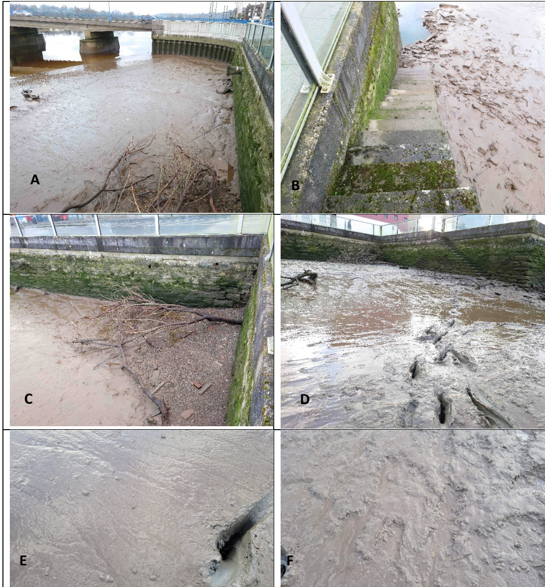
Figure 2 (A) General overview of the site from behind the JFK Memorial. (B) Access steps at southern boundary, also showing mud-covered rubble. (C) Gravel, brick and other debris in south east corner of site. (D) View of algae-covered quay wall from river side. (E) View of the sediment surface along the low water edge of the mudflat. (F) View of the sediment surface along the mid shore level of the mudflat.
