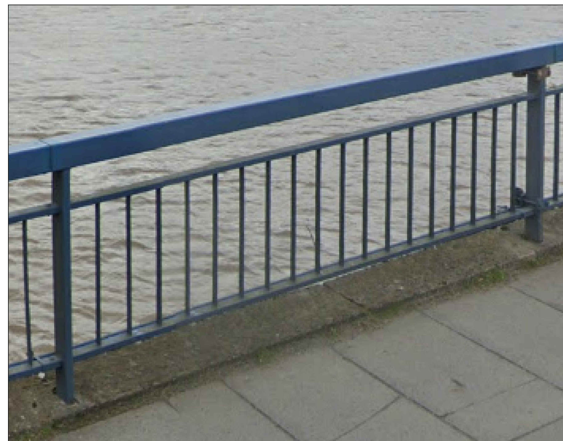
EXISTING PARAPET SAMPLE
