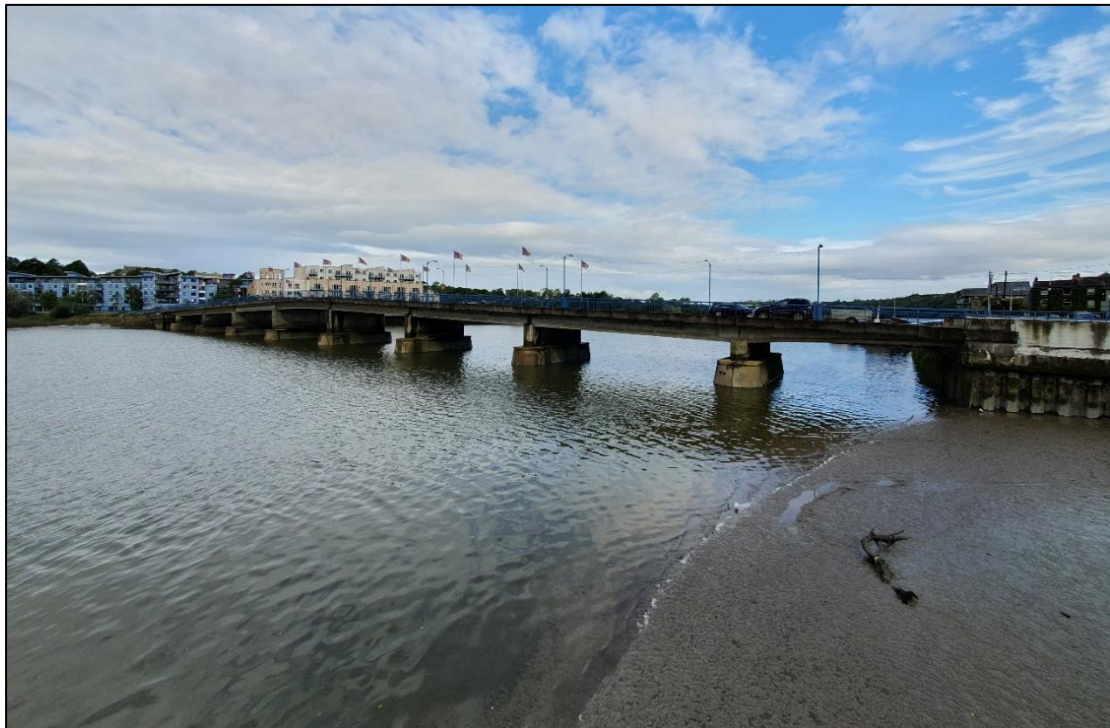
Plate 2-7 Estuary / Tidal River flowing under O'Hanrahan Bridge.
