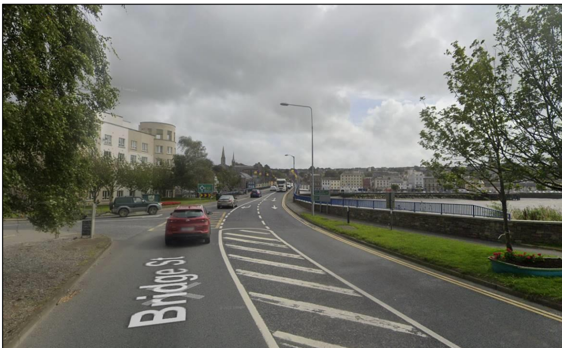
Plate 2-4 Rosbercon Quay with view to the east. The proposed development will provide a connection to the South – East Greenway that will be part of the existing road in the foreground. In the background is the O'Hanrahan Bridge. © Google Street View
