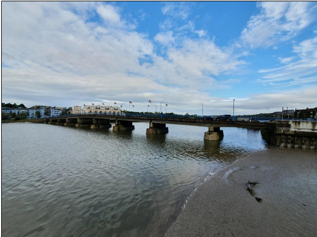
Plate 2-7 Estuary / Tidal River flowing under O'Hanrahan Bridge.
