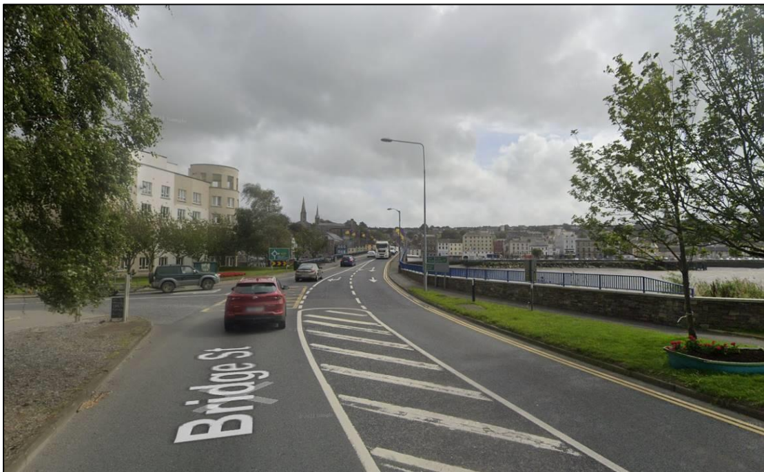
Plate 2.5 Rosbercon Quay with view to the east. The proposed development will provide a connection to the South – East Greenway that will be part of the existing road in the foreground. In the background is the O'Hanrahan Bridge. © Google Street View
