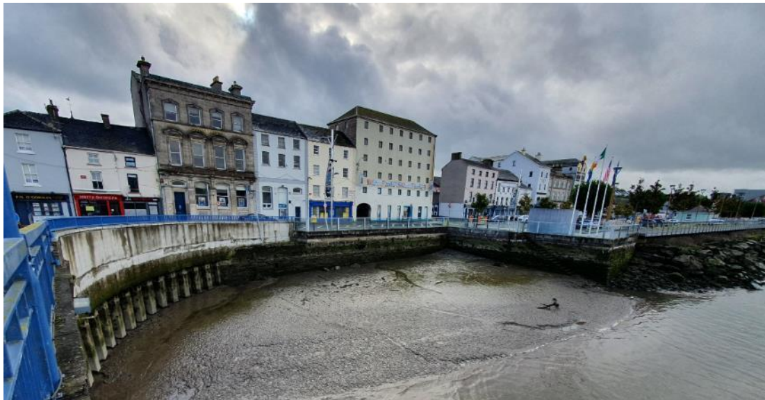
Plate 4.3 Showing the existing flood walls on the New Ross quays
