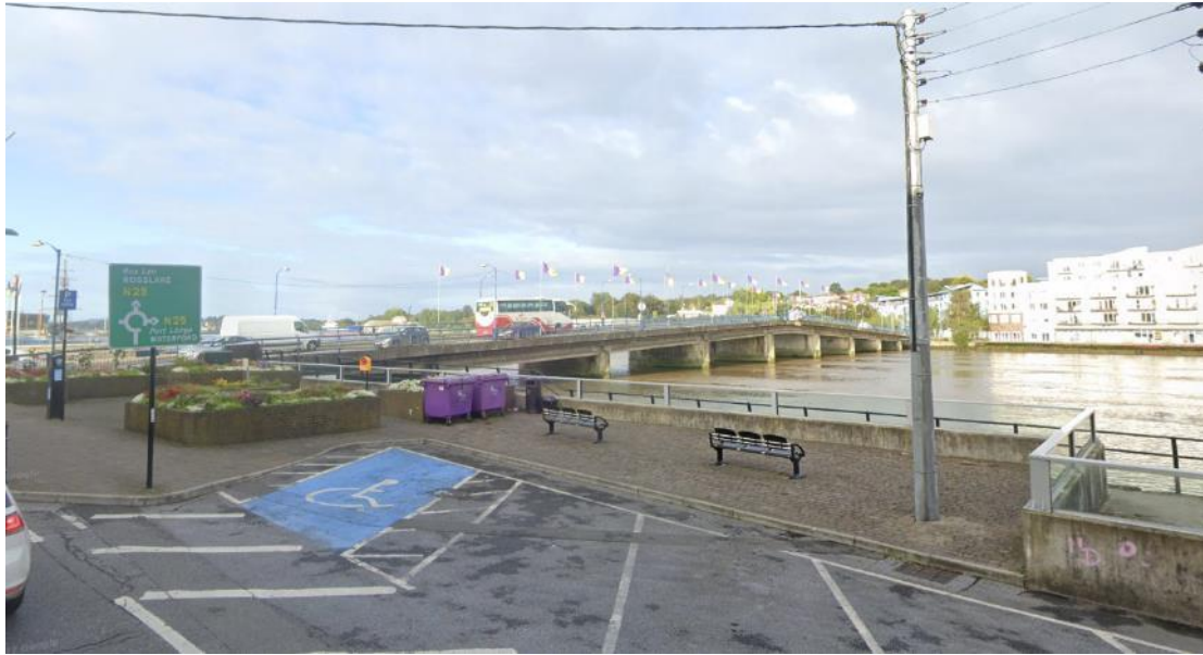
Plate 2.4 New Ross Quay with views to the south. In the foreground are the existing road, parking spaces, existing flood defence wall and a public realm consisting of a small square with benches and flower beds. In the background is the O'Hanrahan Bridge and the Rosbercon Quay. © Google Street View
